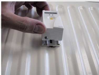
7-14 MOUNTING EURISII ON HEAT CONDUCTOR
