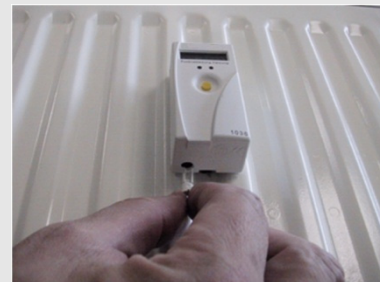
7-15 INSERTING THE SEAL
